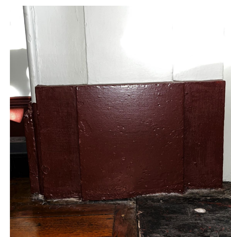
EXISTING PILASTER TO PLINTH DETAIL
