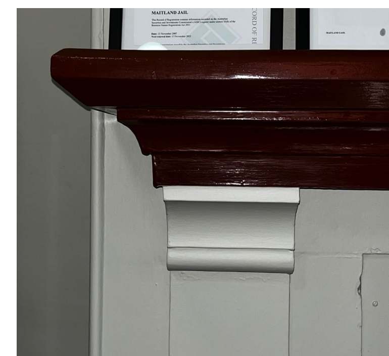
EXISTING MANTEL, CORBEL & PILASTER DETAIL
